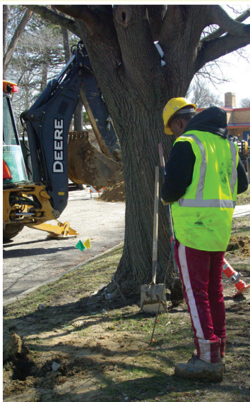
▲ Replace lead service lines in Flint, Michigan.
